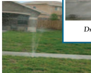
Misdirected sprinkler head
