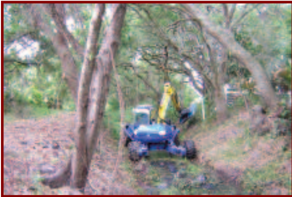
A spyder cleaning ditches
