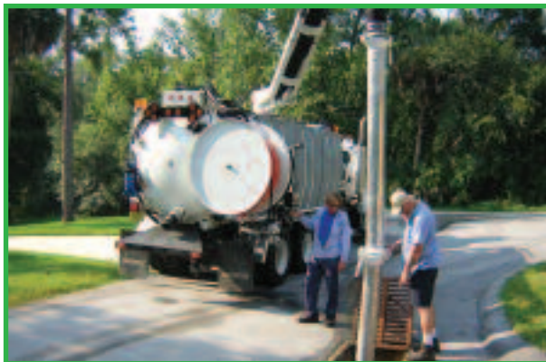
Vac truck cleaning pipes
